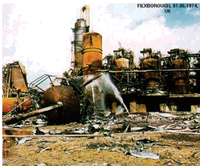
Figure 2. Site of Flixborough explosion (1974).
